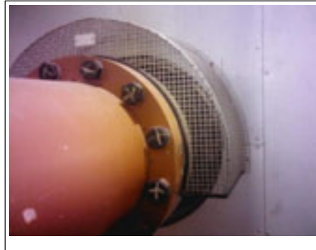
Figure 8: Scene overview. Flange partly protected by mesh for safety reasons
